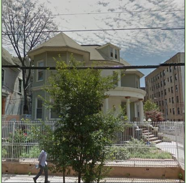
Relevant architectural details include asymmetric façade; unique, semi-circular porch; octagonal tower with turret; dormer windows.
